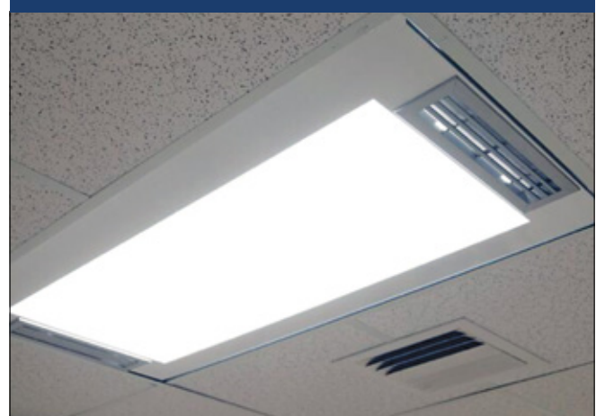
FIGURE 2. UV-C unit installed
