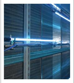
Level 1 – HVAC system efficiency: UV-C energy eliminates and/or prevents the buildup of organic material on the surfaces of cooling coils, drain pans, and interior duct surfaces. This improves airflow, returns and maintains the heattransfer levels of cooling coils to "as-built" conditions, and reduces maintenance.
